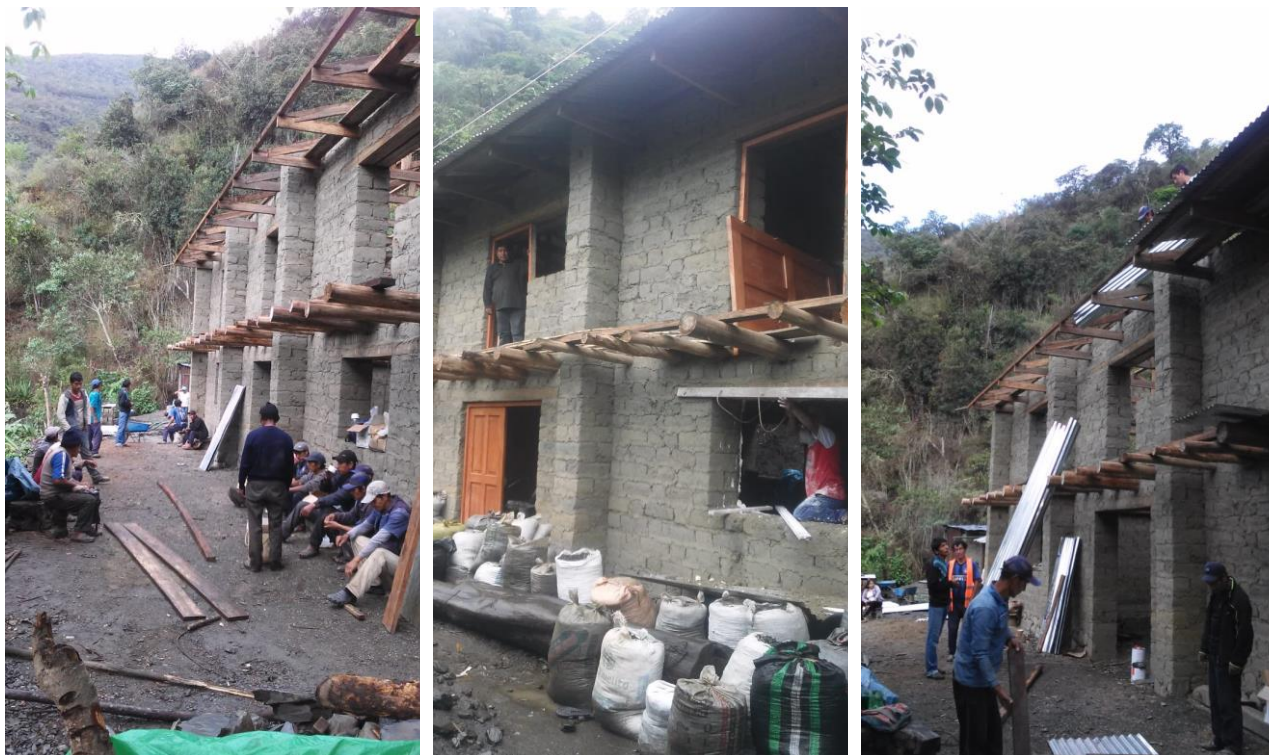
Constructing the community building, which was 80% finished by February 2021
